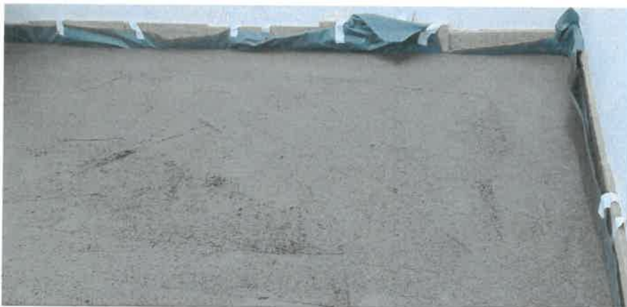
Figure 2: installation situation of floating cement screed
